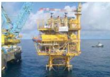
Figure 2. Installation of PBKUM topside, Gulf of Mexico.
